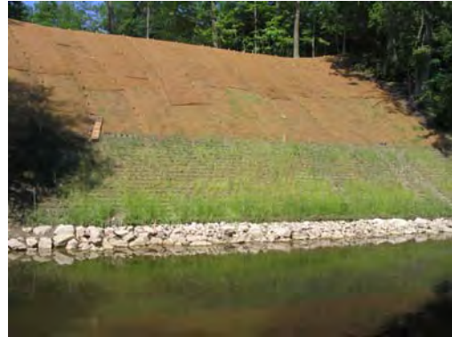
Figure B-4: Rock toe, stacked geocells, and fabric at hart Park, Milwaukee.
