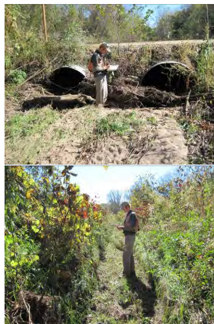
Figure C-2: Etter Creek, Reach 2 (Top) Stn 4,050 looking downstream undersized culverts under Ravenna Trail; (bottom) Stn 5,500 looking upstream at straightened channel.
