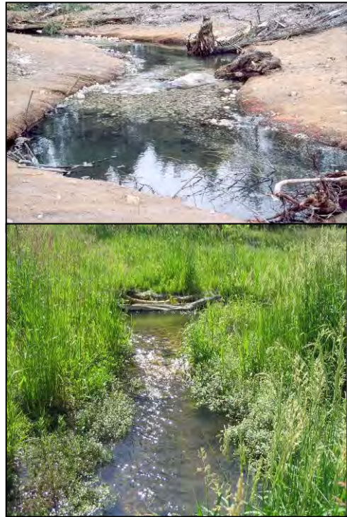
Figure B-1. The above photos show a riffle-pool channel (A) just after and (B) 2 years after construction. Grade controlling riffles can be built either in conjunction with armored banks to prevent channel migration, or with sediment input in mind, so that as the stream moves laterally, new riffle lobes will form (photos Inter-Fluve).
